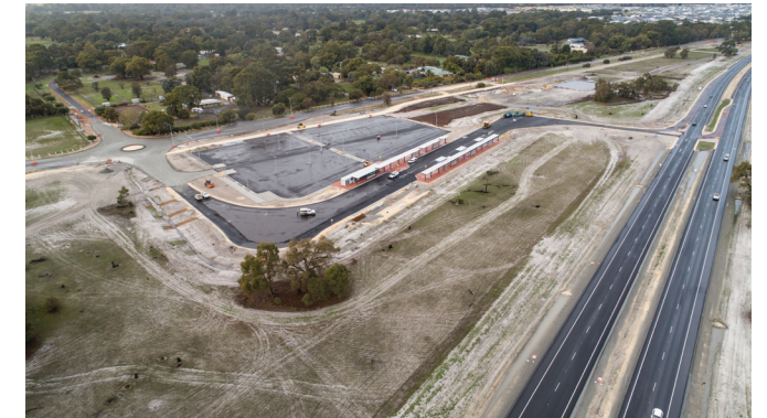
Henley Brook and Henley Street roundabout progress works
