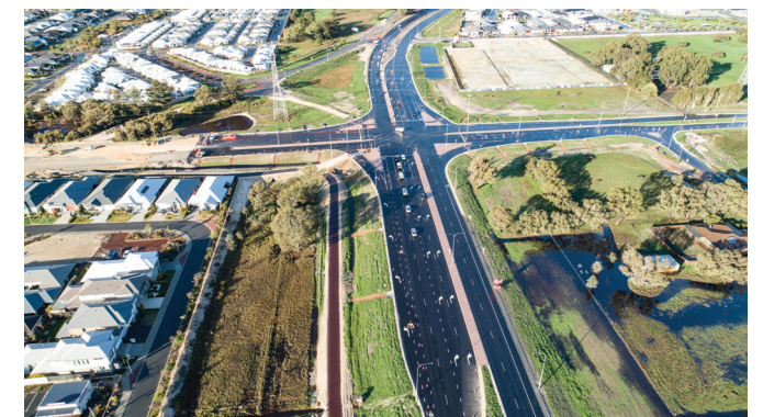
Marshall Road intersection looking south to Reid Highway
