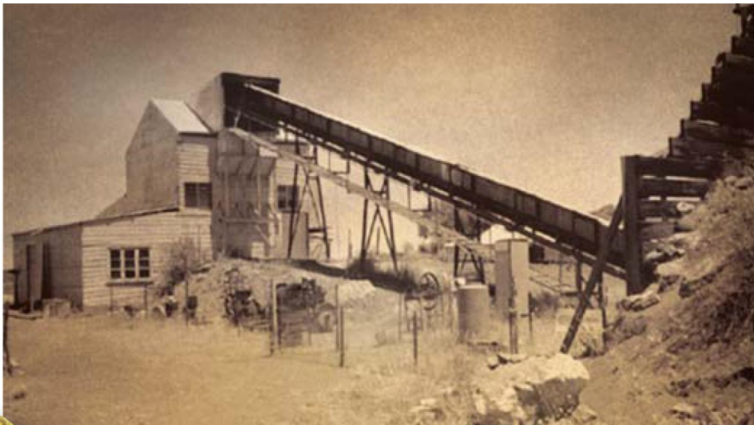
Paynes Find Battery – built in 1911 – now a museum structure
