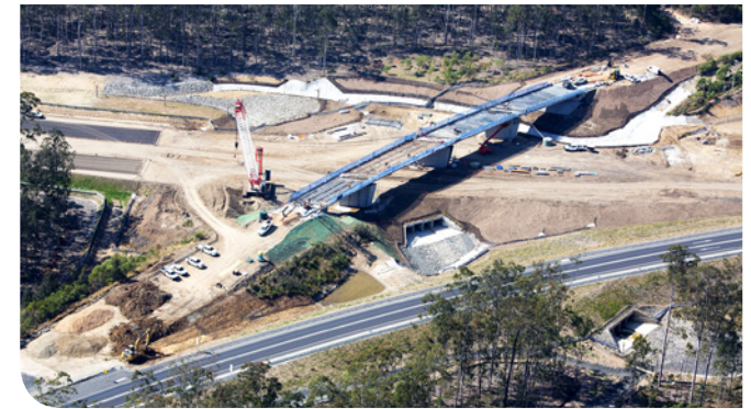
Bridge work continuing as part of the Glenugie South interchange
