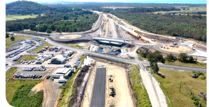
Aerial view of the Broadwater interchange looking north-east
