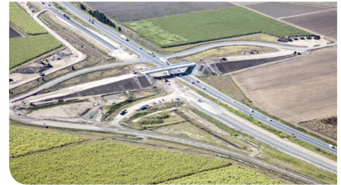
Aerial view of Chatsworth Road South overpass bridge
