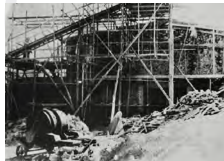
Construction of the old gymnasium, music, geography and art rooms
