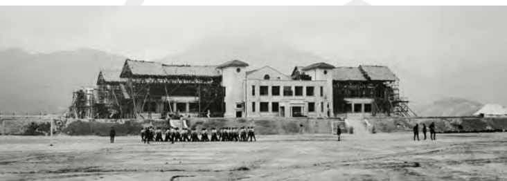
Construction of the third storey of the DBS main building
