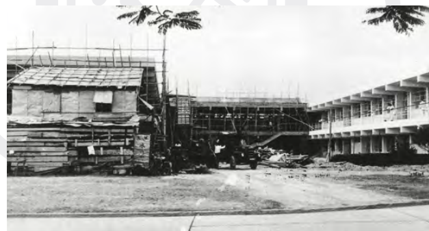
Construction of the New Wing
