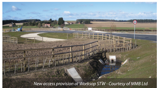
Worksop Sludge Treatment Facility viewed from new access road Courtesy of MMB Ltd
