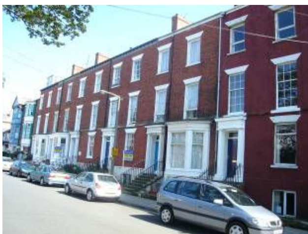
West Terrace, West Avenue Listed but not currently in the Conservation Area
