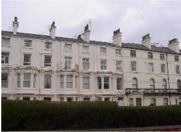
The Crescent – recessive roof with Visually strong chimneys which Contribute to the architectural rhythm
