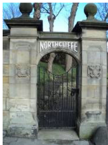
Listed gates to Northcliffe
