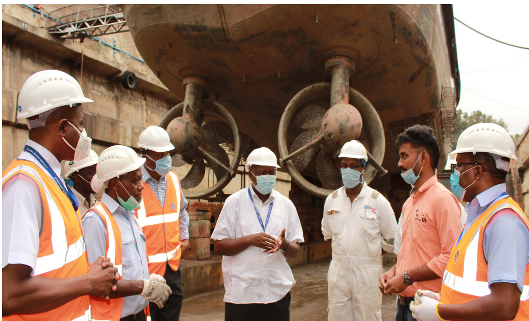
KPA team of marine engineers and other officials inspect on-going works on tug boat DUMA II at the African Marine and General Engineering (AMGECO) dry-dock.
