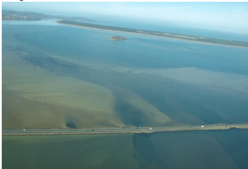
Figure 6.7: Aerial oblique image of 2 nd causeway showing tidal channels draining from Orielton Lagoon through culverts and pipes. (Source: image I.Houshold May 2009)
