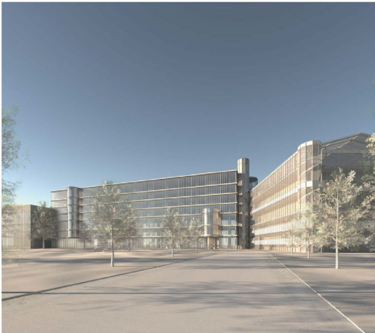
A winter sun brushes over the new (IT) building. The volume provides a clear orientation, and it discloses the strong identity.
