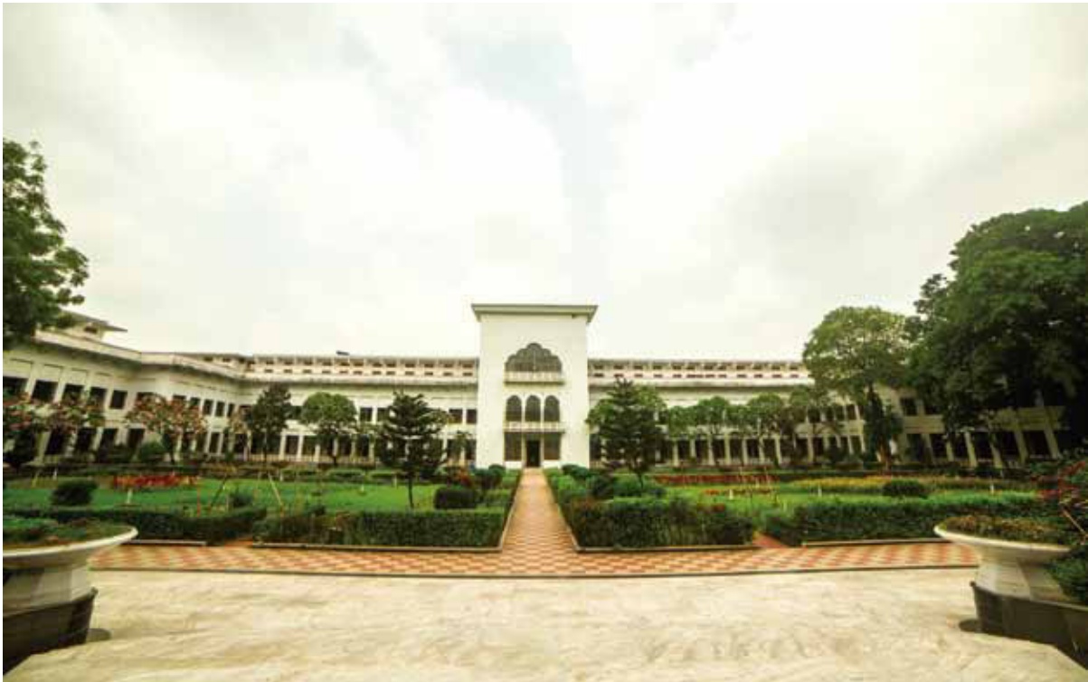
Inner garden of the Main Building of the Supreme Court
