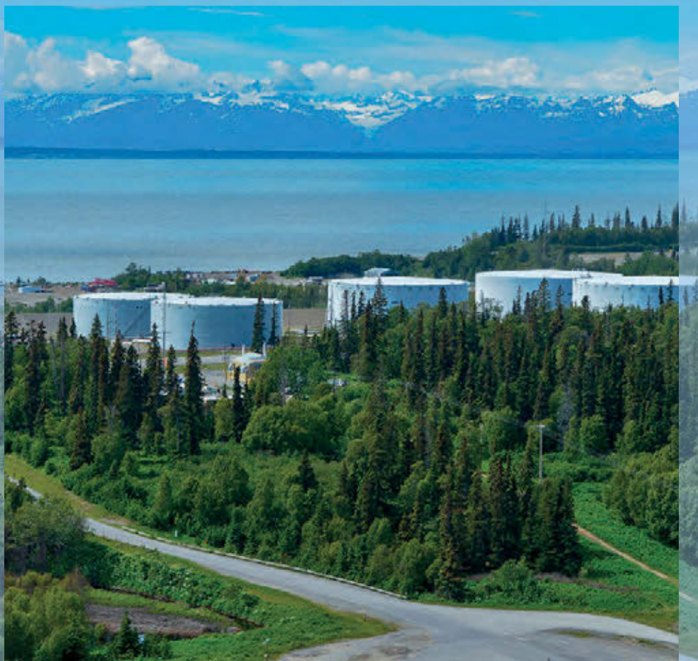
Bulk storage at Kenai refinery in Alaska
