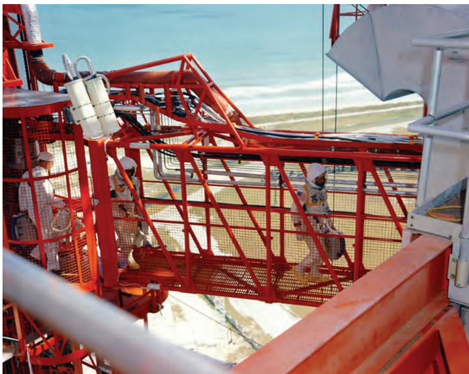
The access arm at Launch Complex 34 where the crew would have demonstrated an emergency escape had the test gone as expected.
