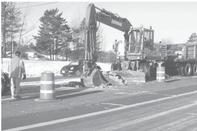
Removing a concrete pavement section in Wisconsin.
