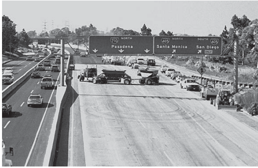
Traffic is rerouted during the long-life asphalt concrete project on I-710.
