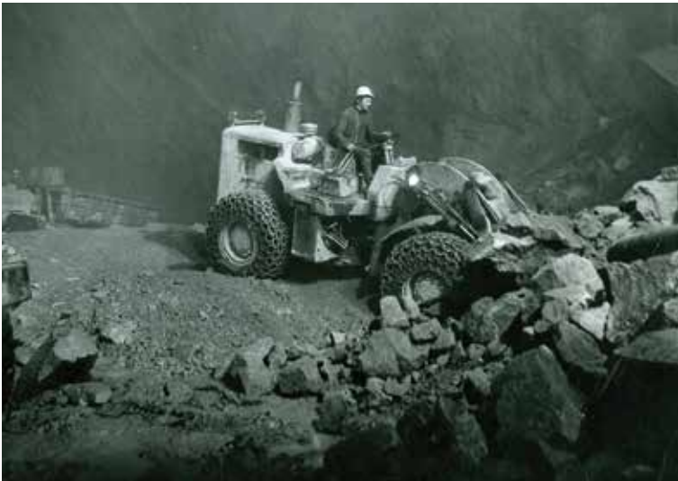
Excavating the cavern, which would house the massive power station
