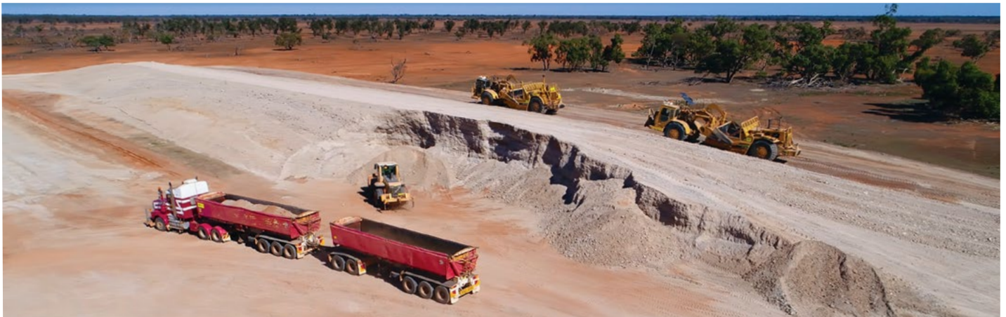
Cobb Highway – road construction
