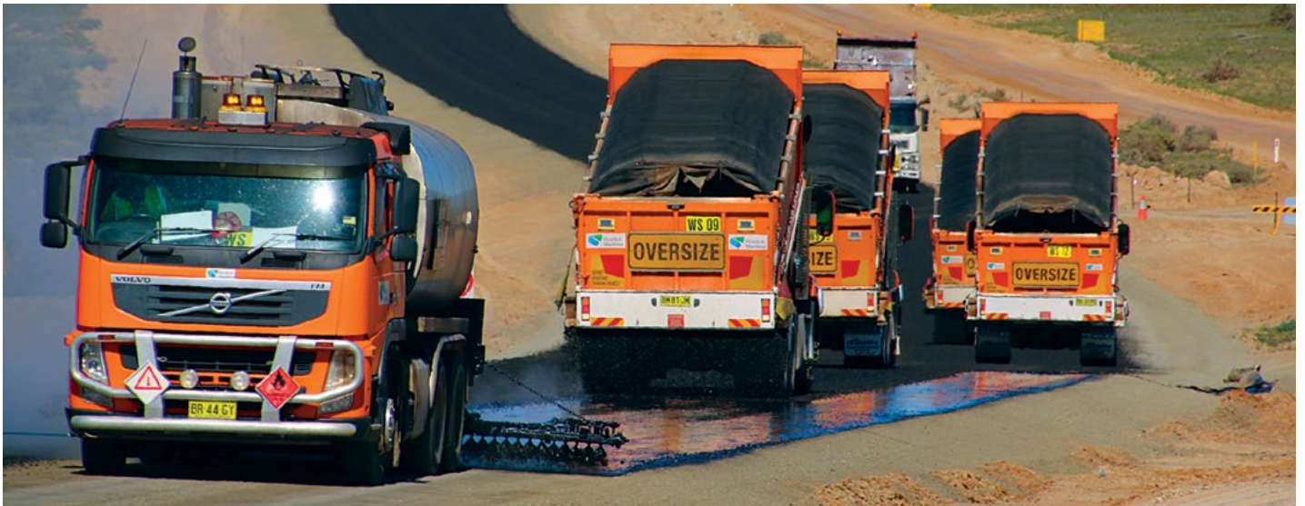
Euriowie, Silver City Highway – placing the new seal on the road
