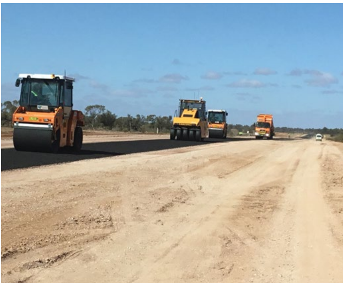
Cobb Highway – sealing work
