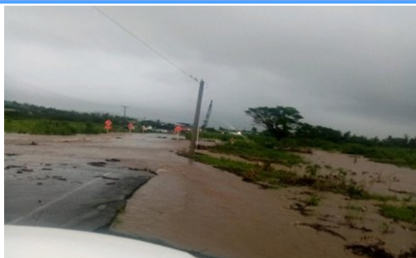
Figure 11: Flooded Kings Road in Tavua on the 13 th . Source: Fiji Roads Authority.
