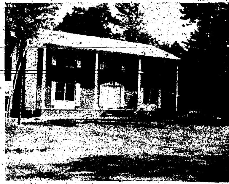
CUSTOM BUILT HOME — Mr. and Mrs. George Bischoff, formerly of 421 Manor Ave., have moved into their newly-constructed colonial home at 94 Belmont Ave., shown above. Mr. Bischoff, owner of Arts and Production Service of 23 North Ave., E., had his home custom built by Anthony Iaiane. The above transaction was negotiated by Mary Knerim of the G. E. Howland office.
