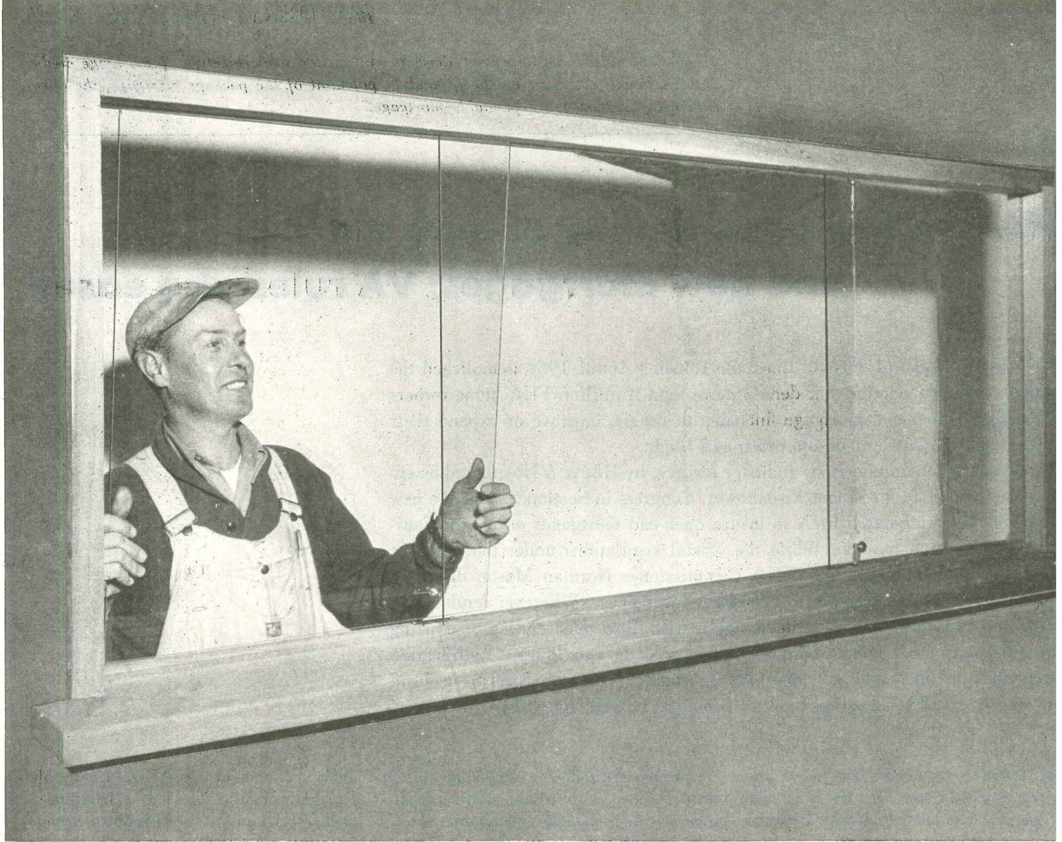
*Glass lifts out for painting or when cleaning. Carpenters and Builders like ease of installation.*
