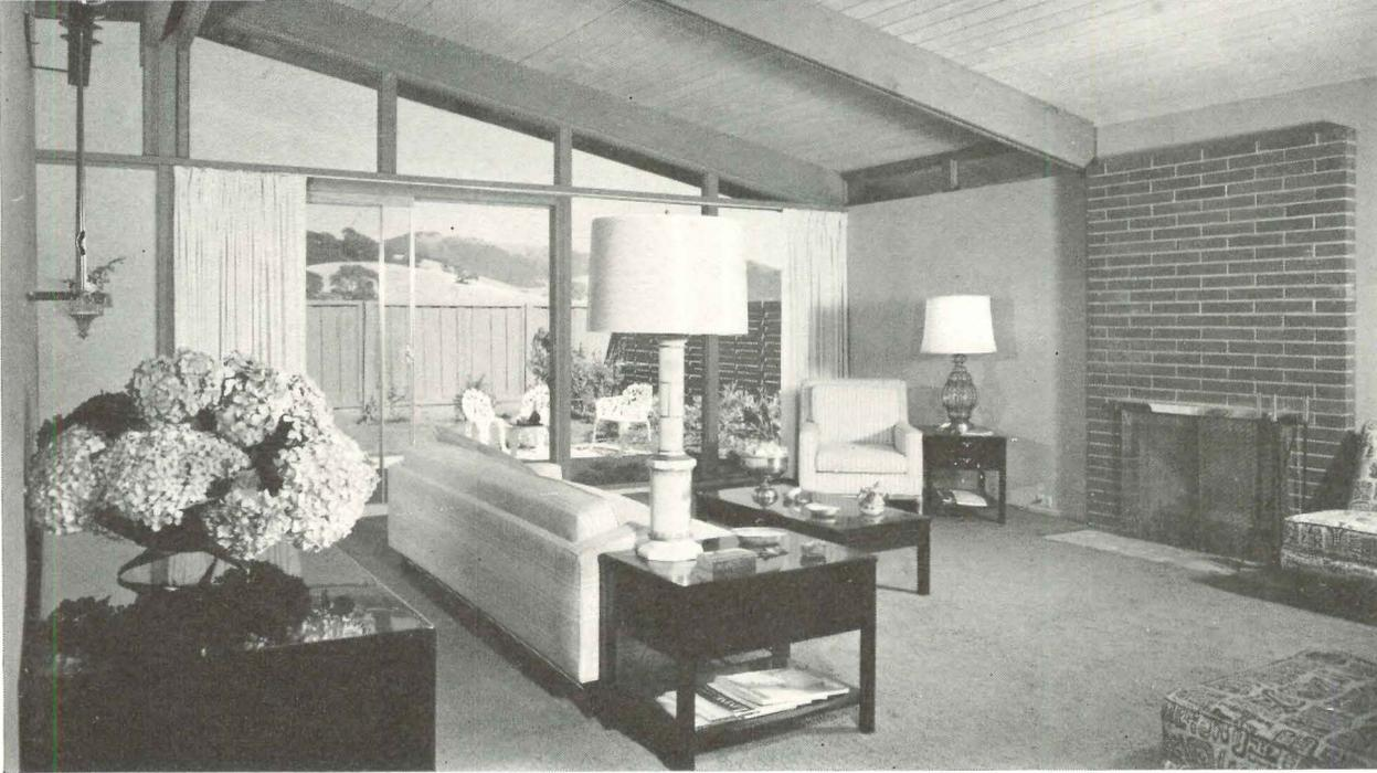
Heavy beams of doug fir 2" x 12"s with plank: T&G 2" x 6"s are characteristic of all Terra Li houses. Over the ceiling is 1/2" of glass fiber, the built-up roof topped with light-colored gravel.
