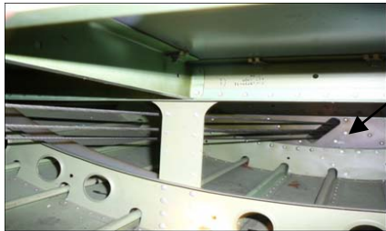
Bulkhead at STA 376.0 (Looking Aft)
