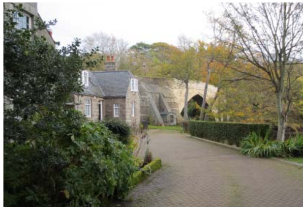
Original salmon house and bridge
