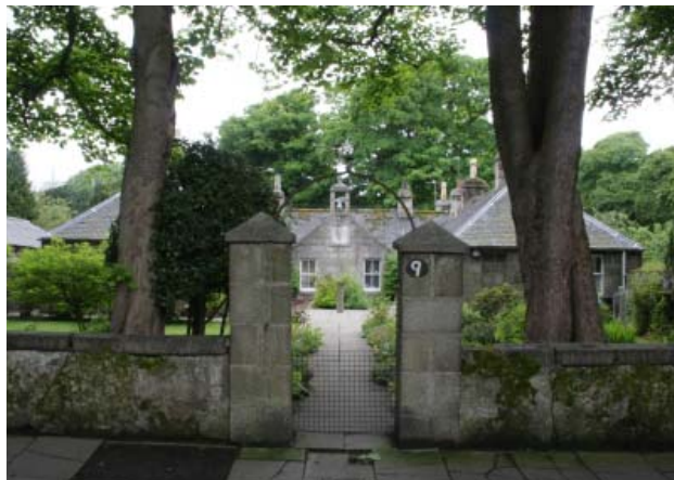
Mitchell Hospital, 9 The Chanonry
