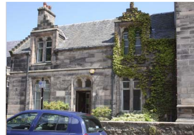
Top: Public convenience and shelter, High Street Bottom: 24 High Street
