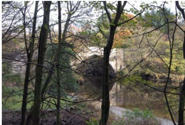
Left: Self-seeded trees obscure views of the bridge Right: Netherdon, The Studios
