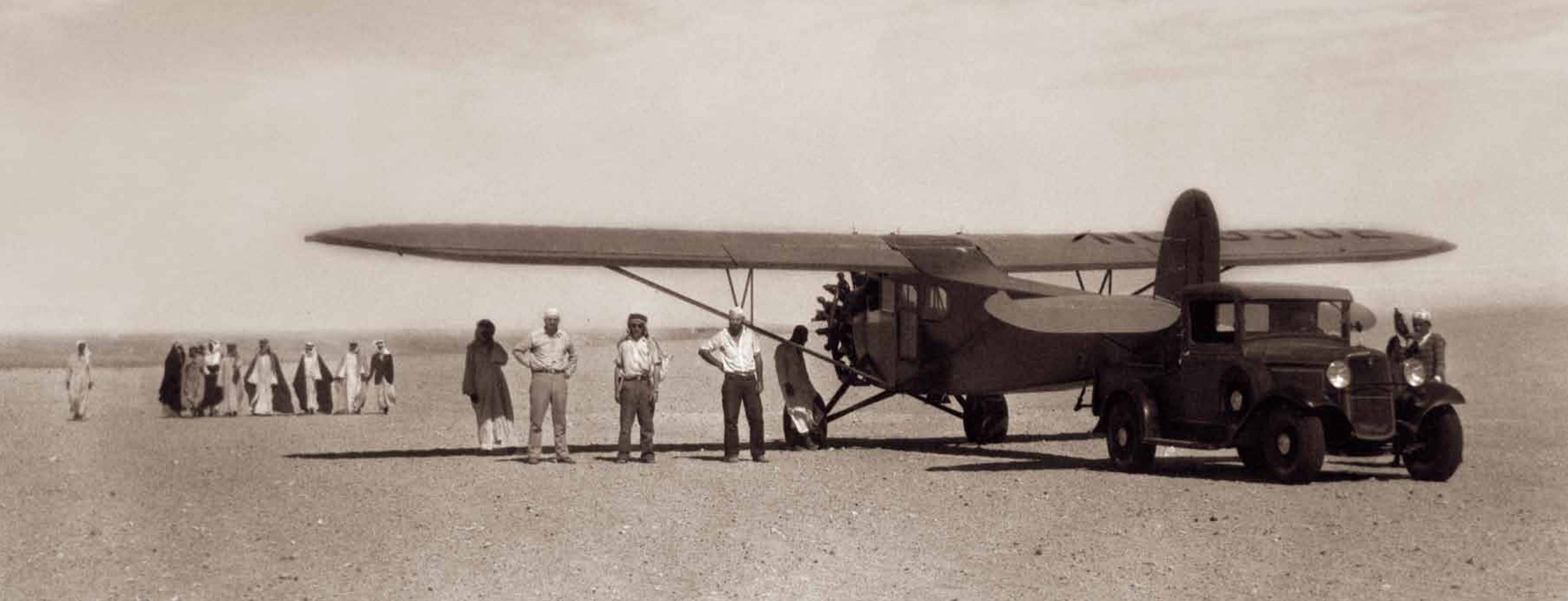
A Casoc pickup truck tows the Fairchild 71 into position for takeoff on a makeshift runway near Jubail in 1934. The aircraft enabled Casoc to map the massive concession area much faster and to supply remote exploration camps, where geologists often stayed for months at a time.
