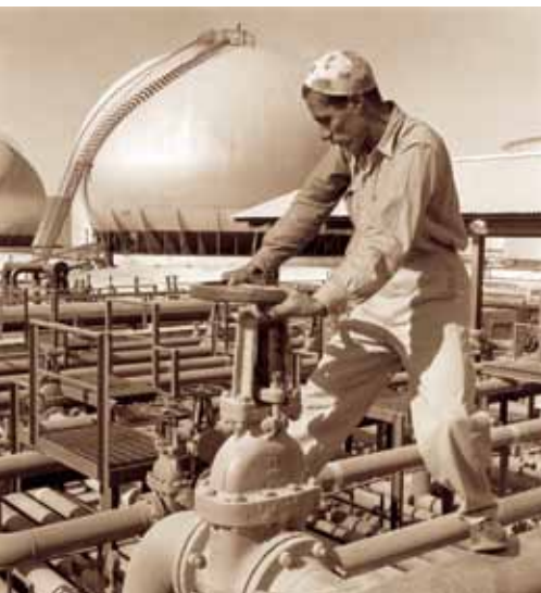
'Id ibn Ahmad opens a gasoline-blending discharge valve at the Ras Tanura blending and transfer pump house in 1956, a year in which the refinery processed more than 70 million barrels of oil, nearly double the amount of 1950.
