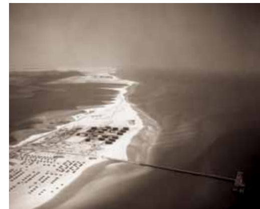
Shown in the mid-1940s, the Ras Tanura Refinery complex spanned the entire width of a narrow sand spit. Rows of tanks stored oil for export tankers calling at the terminal.
