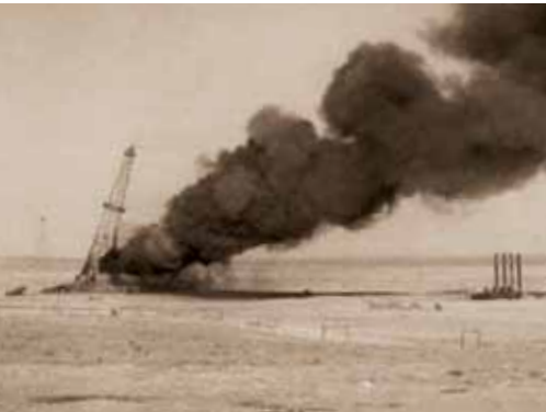
The fire at Dammam Well No. 12 on July 8, 1939, burned so hot that the 41-meter-high derrick collapsed after roughly 10 minutes. Five men, four Saudis and one American, died in the blaze. Casoc crews, working with limited resources, improvised a solution to cut the flow of oil feeding the fire.
