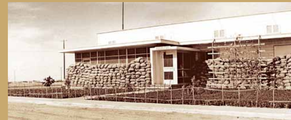
Facilities such as the Dhahran hospital were protected by sandbags during the war years. Casoc also built heavy masonry walls around key installations in Dhahran and the main refining area of Ras Tanura Refinery.
