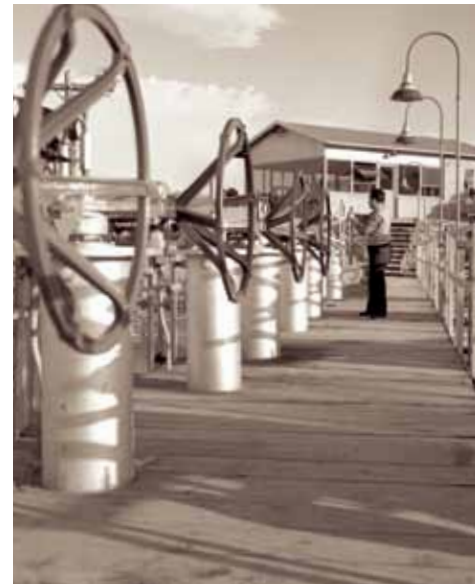
A worker adjusts a valve at Tapline's Sidon, Lebanon, terminal where the first tanker arrived December 2, 1950. In 1951, its first full year of operations, the Sidon terminal received 14.2 million barrels of oil from Tapline. Seven years later, the figure had risen to more than 135 million barrels.
