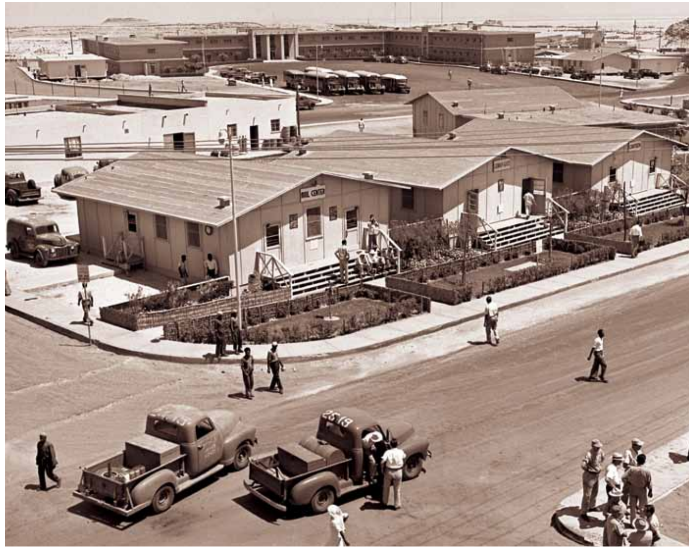
The heart of the Dhahran community is this row of three buildings, which house a canteen, post office and laundry. The company's headquarters offices rise in the background of this 1952 photograph.
