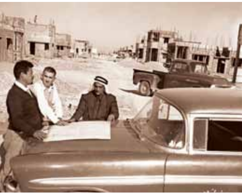
Surrounded by the half-completed homes of the Madinat-Abqaiq development, Ralph Tufley, from Aramco's Home Ownership Program, meets with contractors Muhammad Al-Khatib and Hamad Abu Nahyah to discuss construction progress in 1958.
