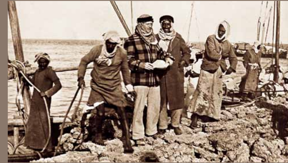
Casoc resident manager Floyd Ohliger, shown wearing a checked jacket, oversees a delivery of furush rock in 1935 that was used to build the al-Khobar pier. To his left is Ahmad “Mussolini” Al-Somali.
