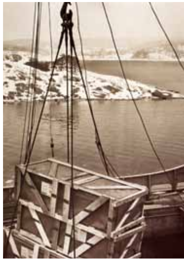
ABOVE Prefabricated housing, bound for Dhahran, is hoisted aboard ship at an icy Scandinavian port in 1952. By accepting payment in kind from its debtor, Aramco was able to both settle the account and provide needed housing.
