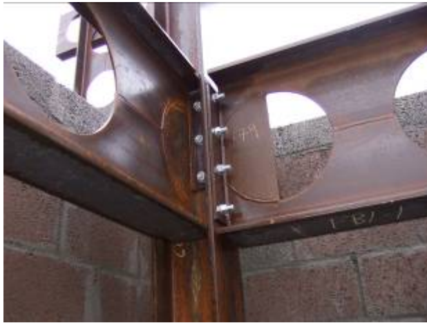
Figure 8-7 : Connection between Beam 2,3 and Column
