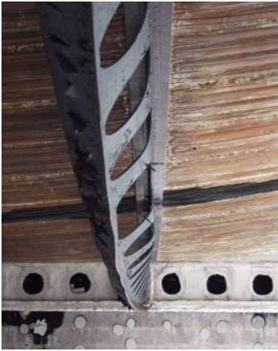
Figure 8-43 : Internal beam near mid span and end connection after fire(Beam 4)
