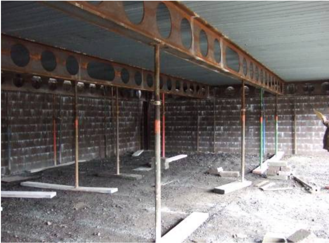
Figure 8-12 : Props supporting beams and slab edges during pouring concrete
