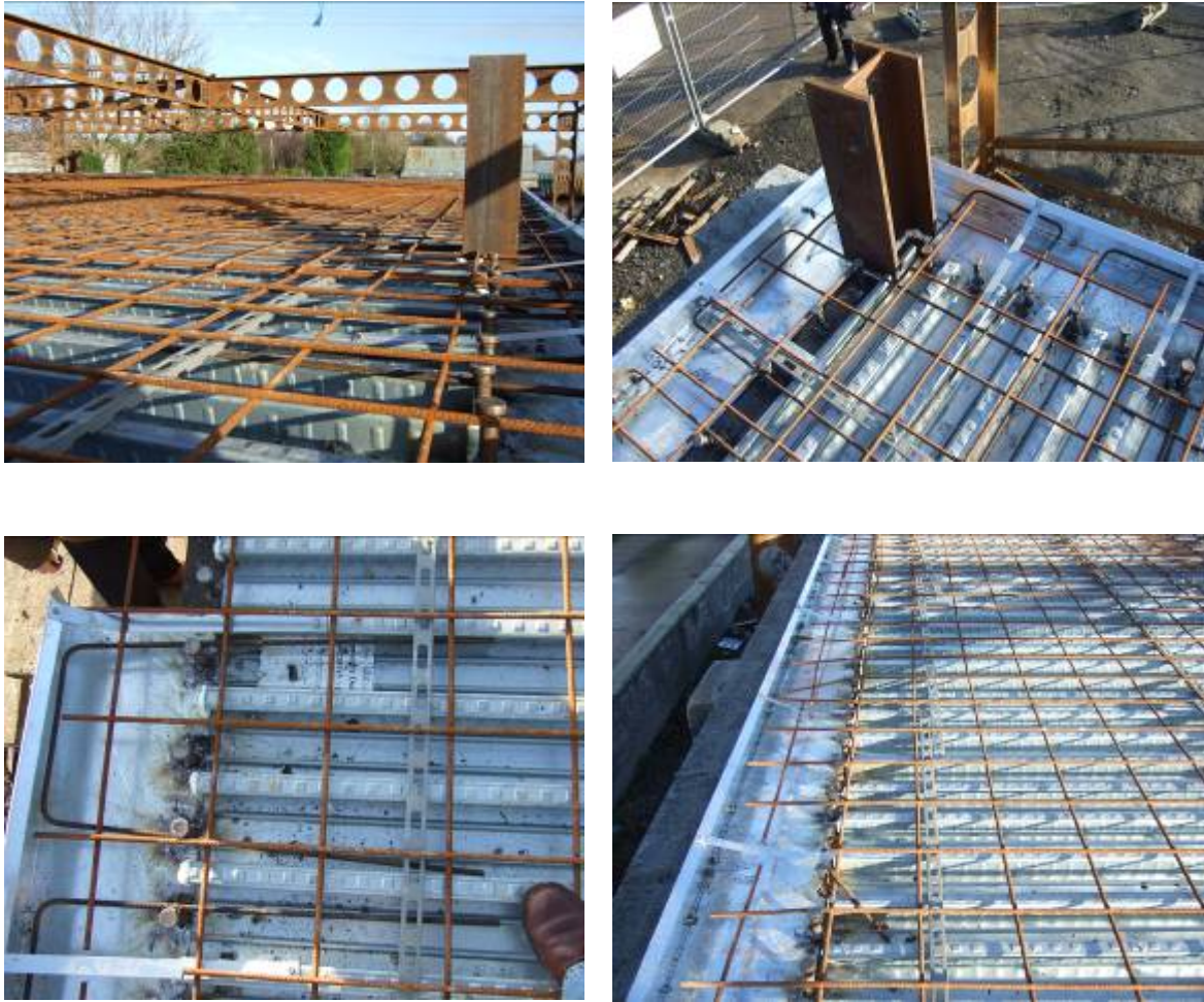
Figure 8–9 : Mesh reinforcement & steel decking before concrete casting
