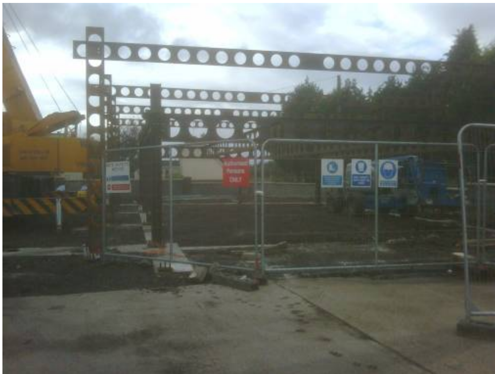
Figure 8-3 : Frame erection
