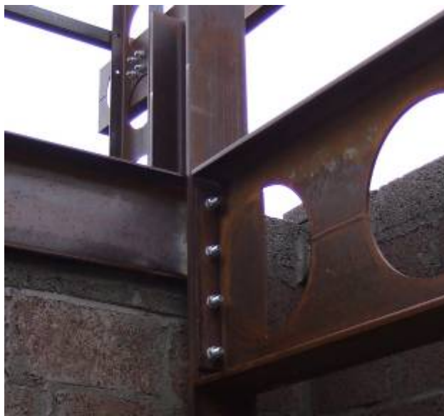
Figure 8-8 : Connection between Beam 1, Column and solid beam
