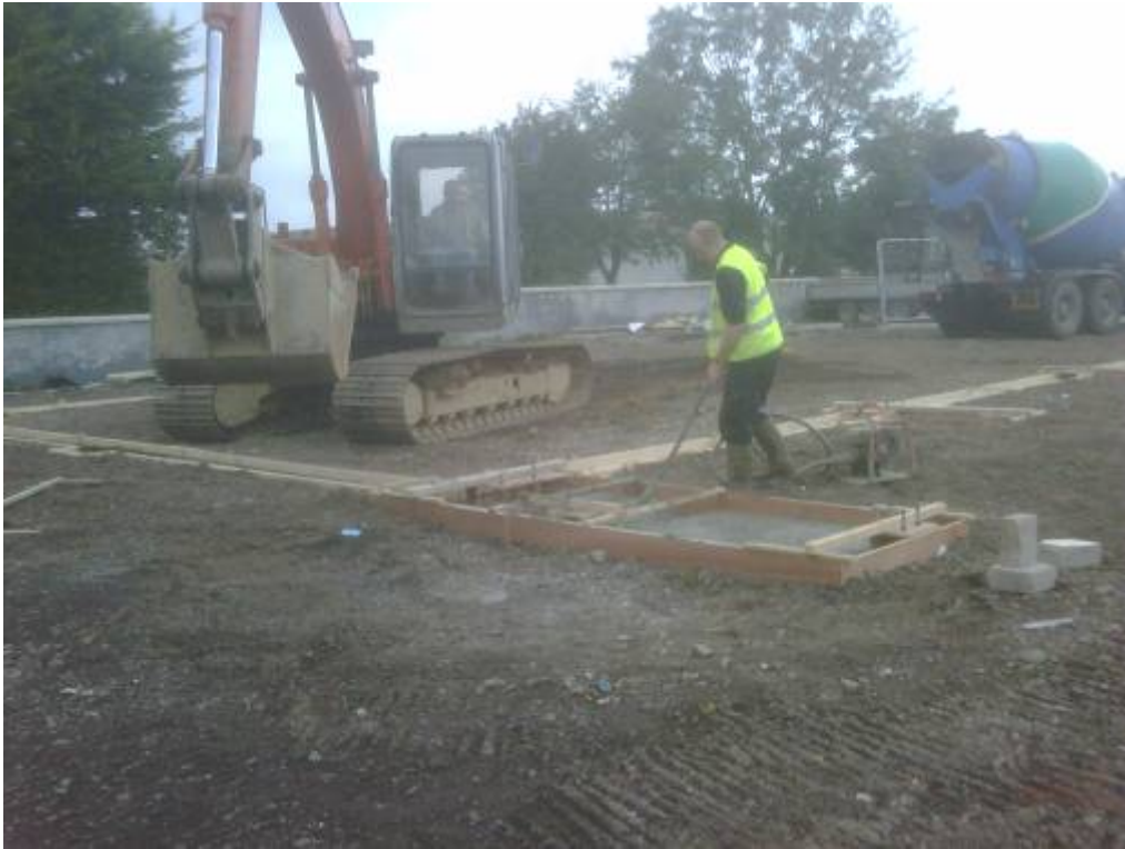
Figure 8-2 : Foundation preparation
