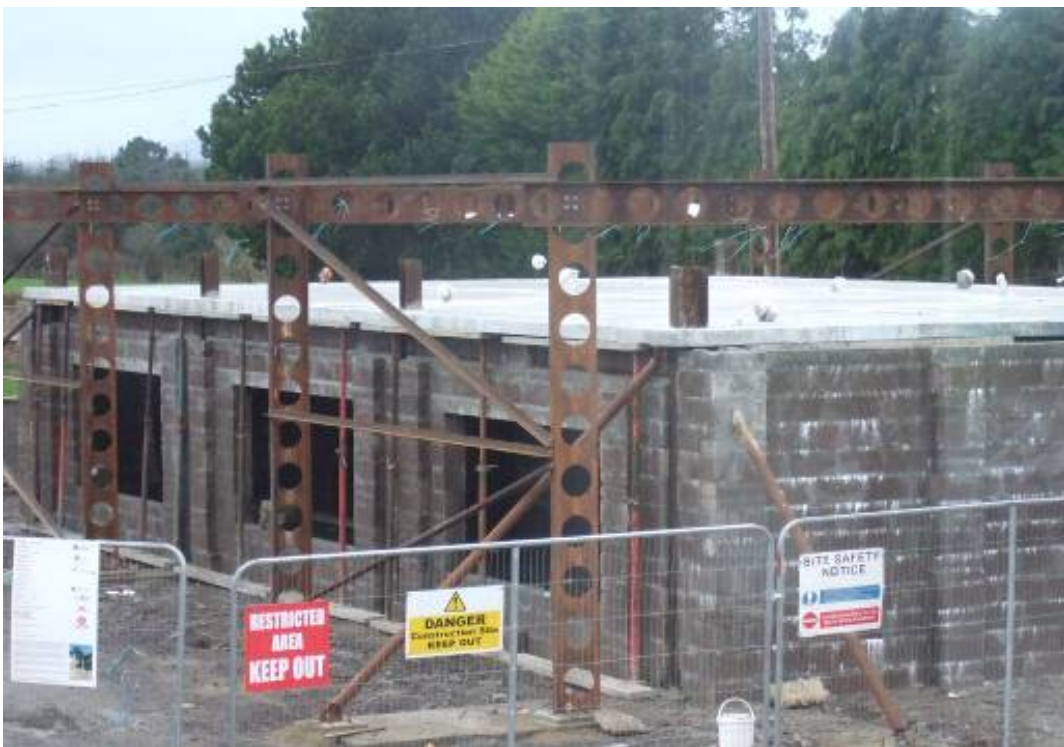
Figure 8-13 : View of the compartment in December 2009
