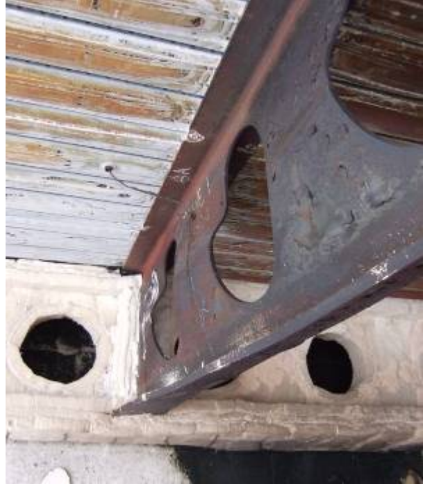
Figure 8-43 : Internal beam near mid span and end connection after fire(Beam 4)
