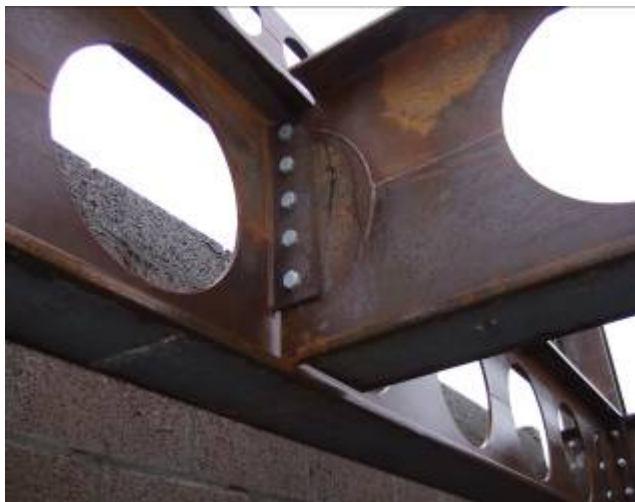
Figure 8-5 : Connection between Beam 2 and 4
