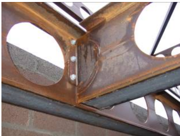
Figure 8-6 : Connection between Beam 2 and 5
