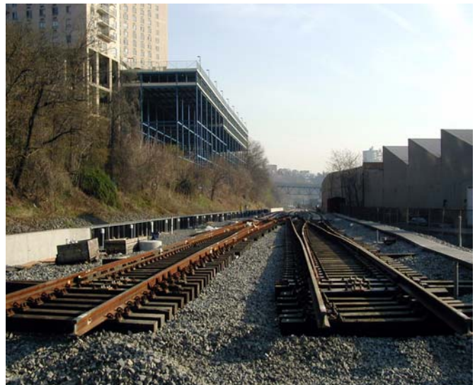
The south end of "Three Roads". This is the 1,700 foot third passing track located just north of 9 th -Congress Station. It is designed for high speed passing (45 mph) of the locals by the express trains, as evidenced by the length of the switchpoint in the Number 20 turnout.
