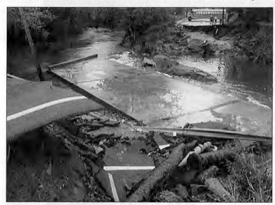
Left: The force of the rapidly moving waters caused the culvert under this bridge to be washed away. Only after the flood waters receded, was the extent of the damage visible.
