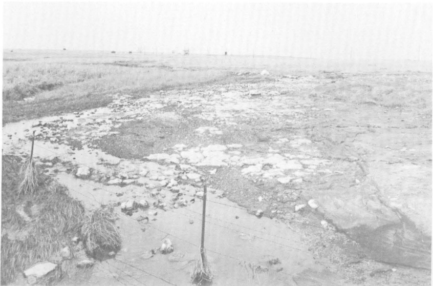
FIGURE 3.—Thin soil mantle over fractured limestone of the Chase Group in sec. 8, T. 25 S., R. 5 E. Mantle permits rapid interchange of ground and surface water.
