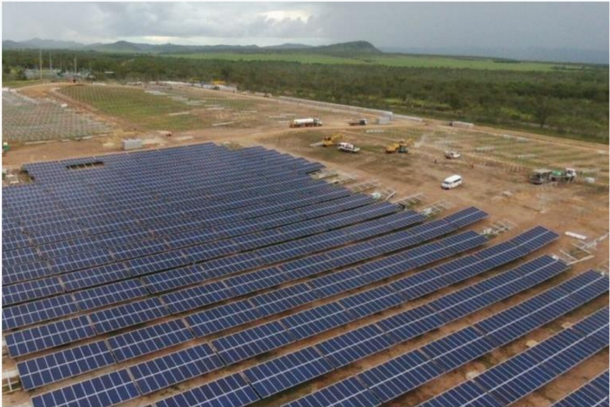
PHOTO: The Lakeland project will comprise 41,440 solar panels and generate up to 13 megawatts of power. (Supplied: Conergy)
