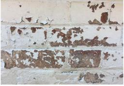
10. Brick laid in a Flemish bond (left) and paint peeling off brick (right), 2018 (BA)
