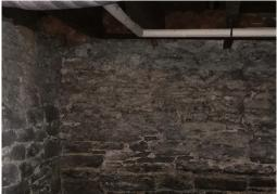
12. Foundation parged and painted on exterior (left), and exterior on interior (right), 2018 (BA)
