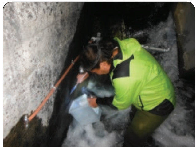
FIGURE 19 // Ngati Hikairo tuna team member Lena Morgan collects elvers at the Otamangakau Valve. The 'attractant flow' delivery pipe is seen to the left on the valve-house wall. (Photo: John Morgan)
