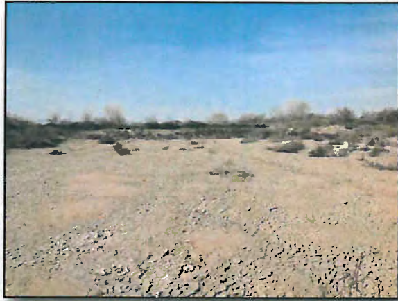
Photograph 11. Looking downstream at Earthen Dam located west of Interstate 5
