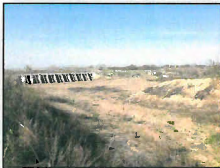
Photograph 7. Looking downstream at Kern River and bike path bridge crossing
