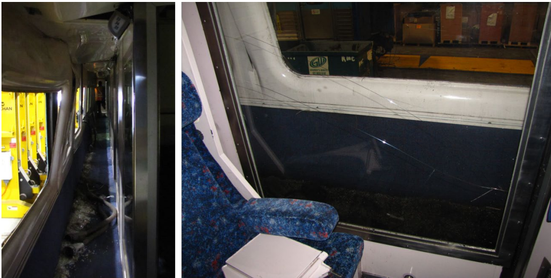
Figure 19: Passenger car A, left-side corridor (left) and fractured glass partition (right)
