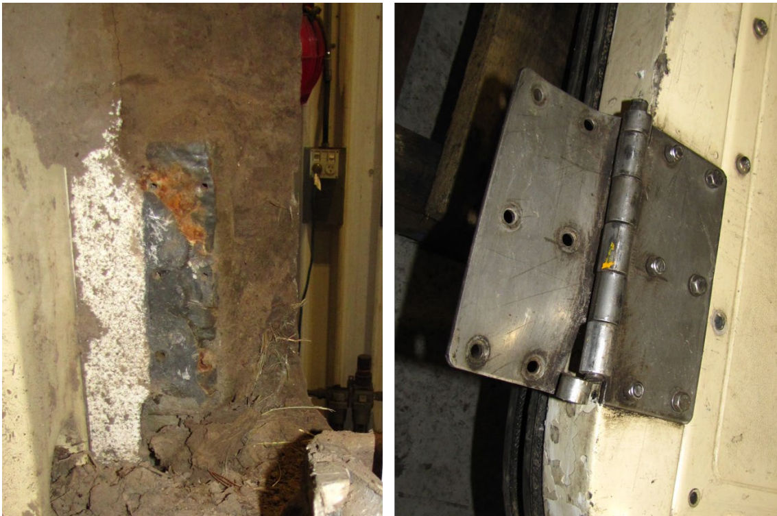
Figure 17: Lower internal hinge of left cab door of XP2018
