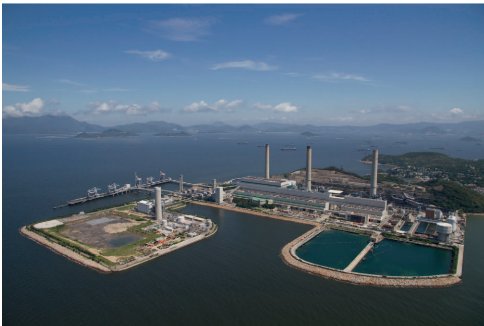
Lamma Power Station
