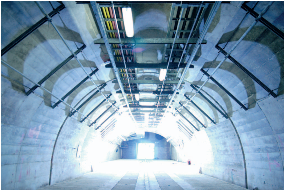
Wah Fu-Bowen Cable Tunnel, the first cable tunnel in Hong Kong
