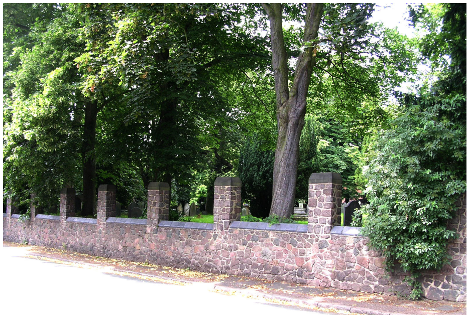
Part of the Mountsorrel granite wall forming the boundary to St. Peter's Churchyard on Vicarage Lane.
