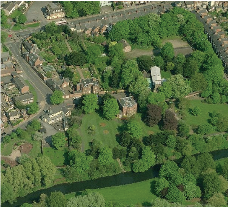
This aerial view from the west shows the significant contribution that trees make to the character of the Conservation Area.
