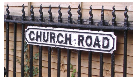
Original cast street sign and wrought iron railings forming the boundary to Belgrave Hall.
