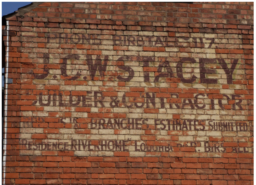
The south-facing gable to 221 Loughborough Road showing remnants of a former painted advertisement.
