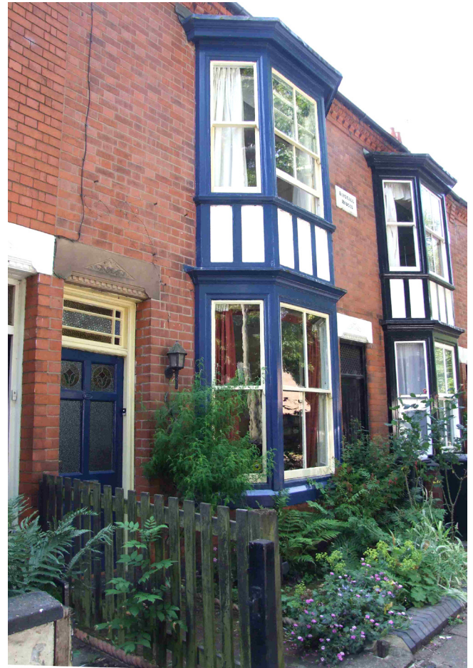
Some of the well-maintained properties in Vicarage Lane with original doors and wooden sliding sashes to the bay windows.
