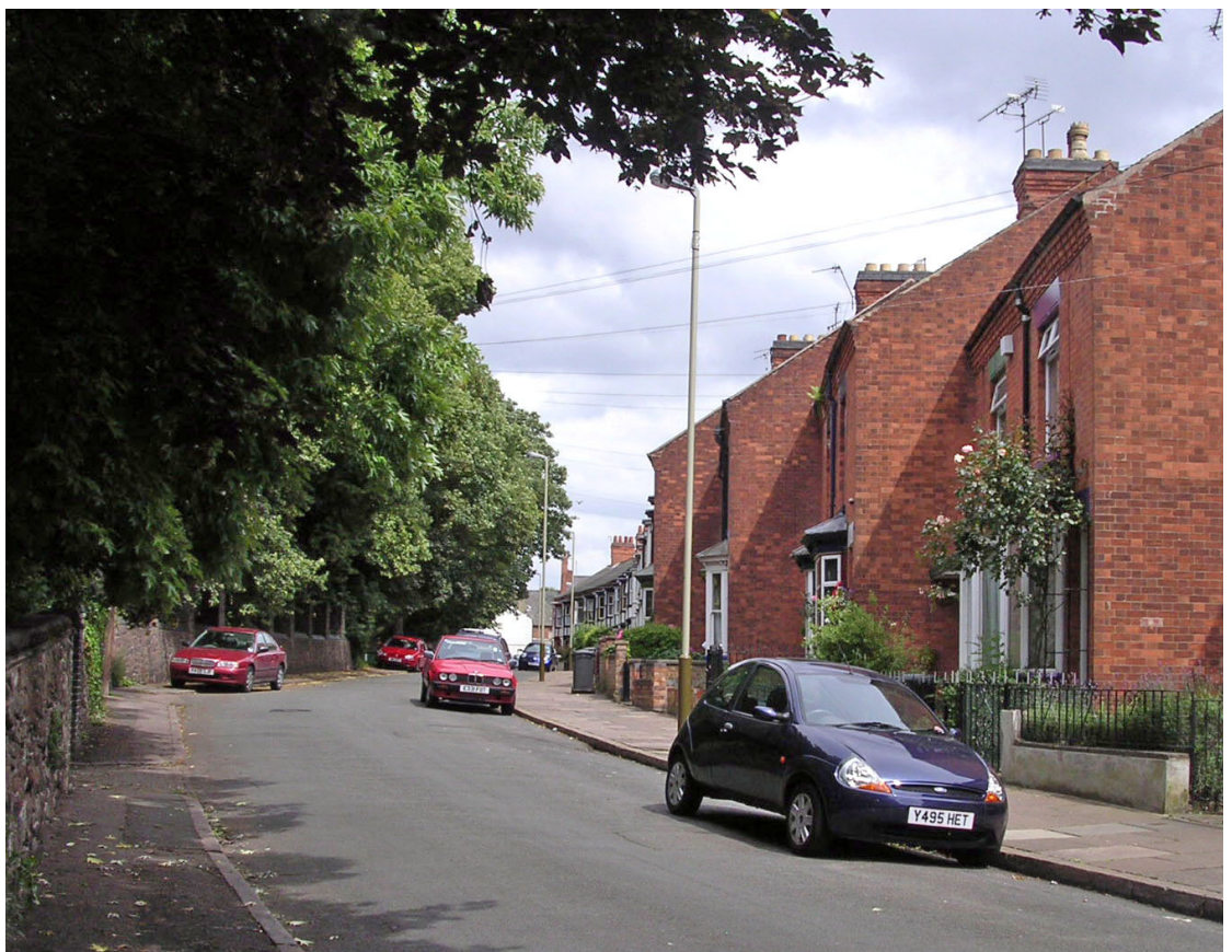
The staggered, curving nature of this row of terraced houses on Vicarage Lane provides a particularly fine piece of townscape within the conservation area.
