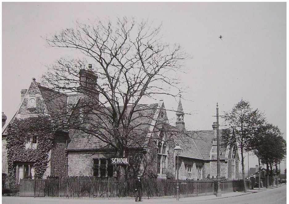
An early image of the former Church of England Primary School at the corner of Loughborough Road/Thurcaston Road. It was constructed in 1887 using local Mountsorrel granite.
