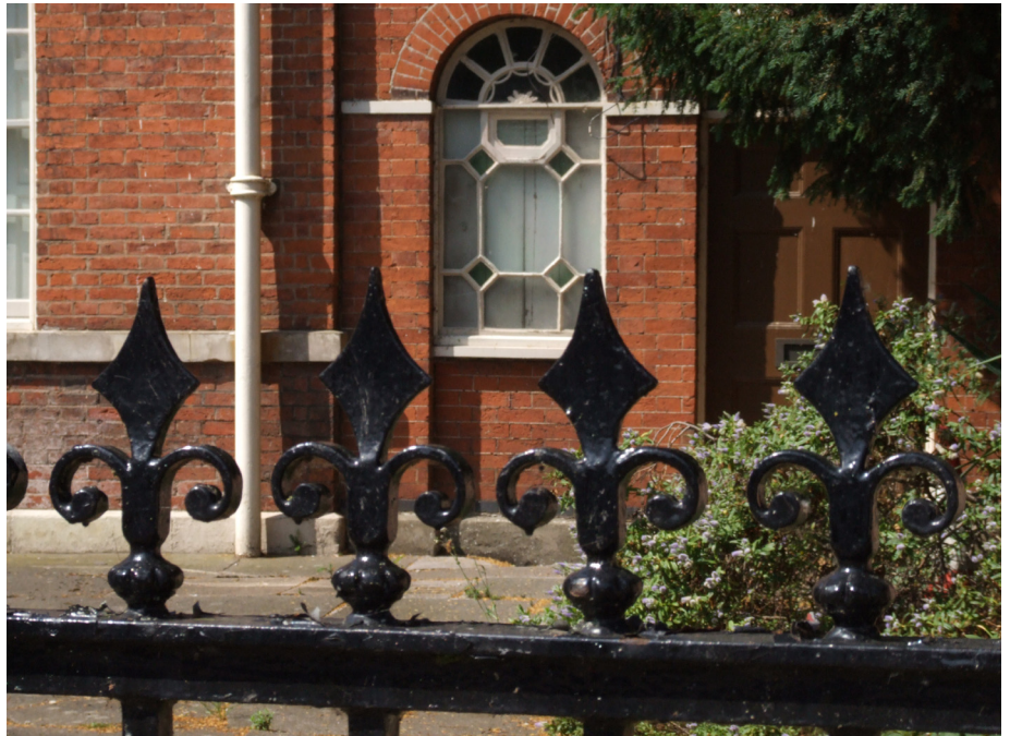
Wrought iron railing details to Belgrave House.
