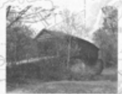
Humpback Bridge Alleghany County
