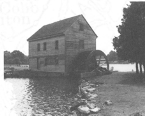
Poplar Grove Mill and House, Mathews County
