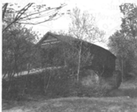
Humpback Bridge, Alleghany County
