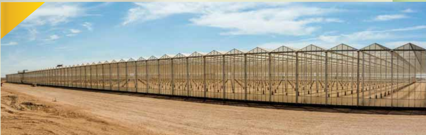
A panorama shot of the Miraah solar energy project
