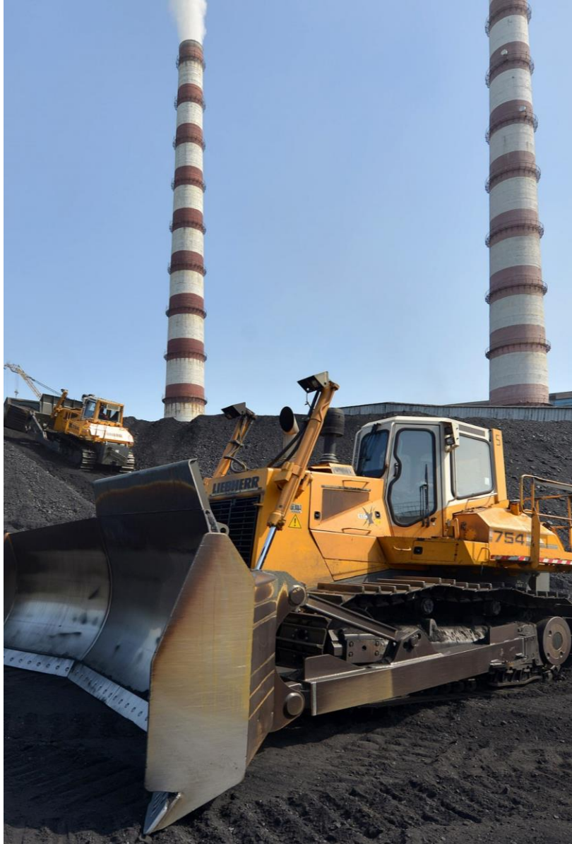
Aksu Power Plant
