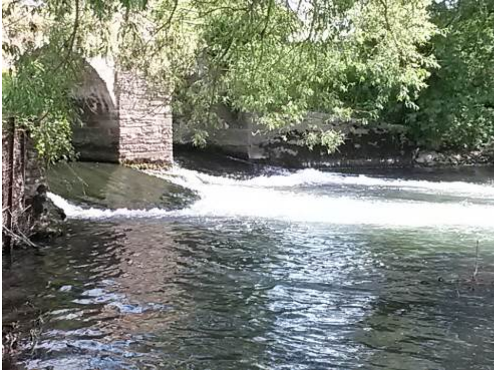
Photo 1 Weir at Eaton Hall bridge.
