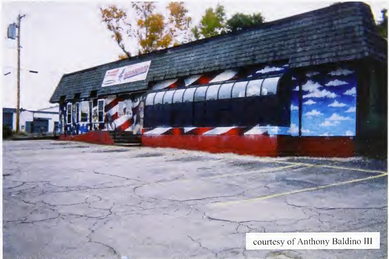
Figure 1-4b. View of the northwest corner showing the sunroom windows [3]
