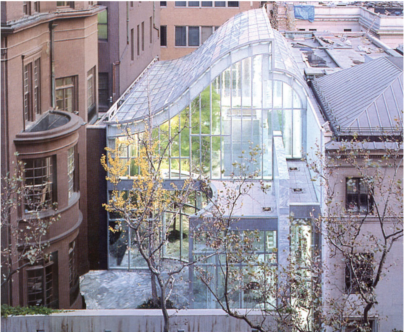
Piano's addition replaces an elegant Garden Court by Voorsanger Architects of New York. Although it was frankly modern, since it was made of veined white marble, limestone, oxidised brass, bronze and seeded art glass, and capped with a graceful piano-curve roof, it met the historic buildings on their own terms and created transitions subtly.
