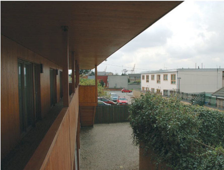
From the upper-level access of the 2003 building, views out across the industrial landscape that surrounds the estate are quite striking. The wooden cladding of this elevation has matured well, as has a sparse amount of planting. It can only be hoped that the newer blocks, one of which can be seen here in the near background, will mature as well.
