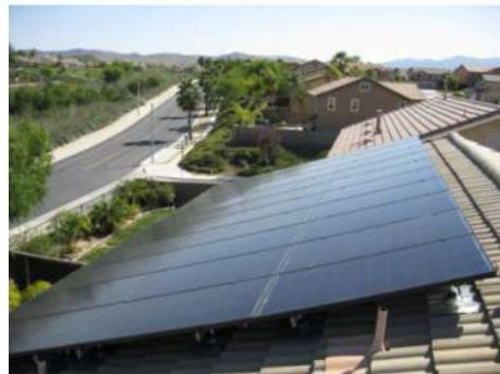
This example was rated a "4" because the array is level and square with cleanly cut rails.
