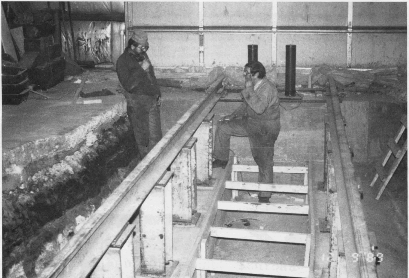
Zeke Fields and Mark Olson discuss the next step in the construction of the LS&M's locomotive pit in the shop.
