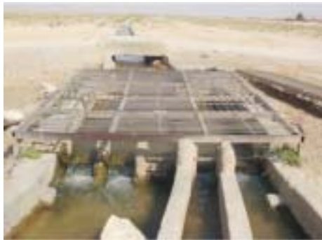
Structure to divide the qanat flow
