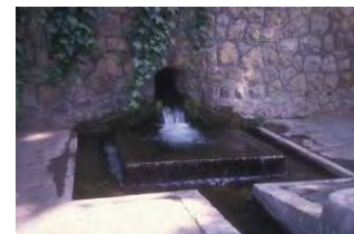
Figure 23 the outlet of a qanat
