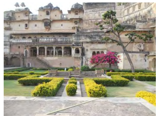
Figure 60 shows the Rawala, queen's resting space meant for leisure. The fort is actually a Rajput fort, but the design is influenced from the Chahar-bagh concept. Built around 17 th century.
