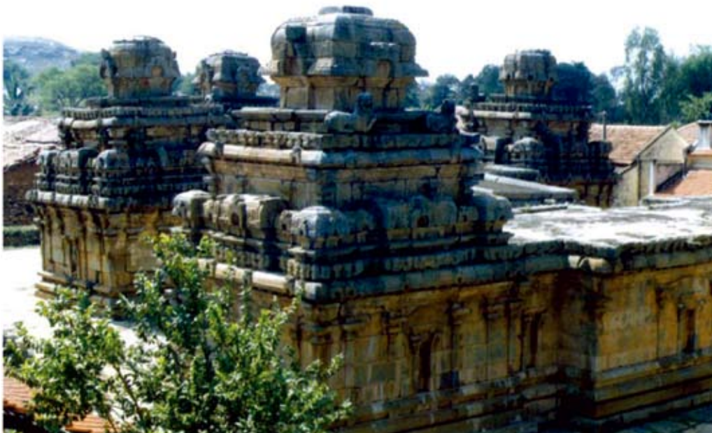
An Aerial view of the Panchakuta Basadi, Kambadahalli
