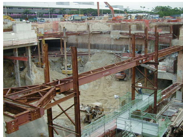
(b) Photograph of Excavation
