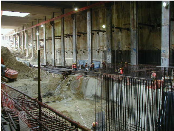
(b) Photograph of Excavation
