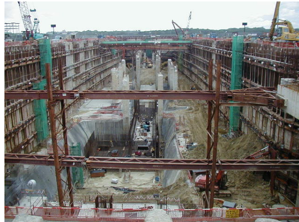
(b) Photograph of Excavation
