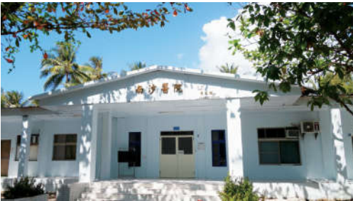
Nansha Hospital on Taiping Island
