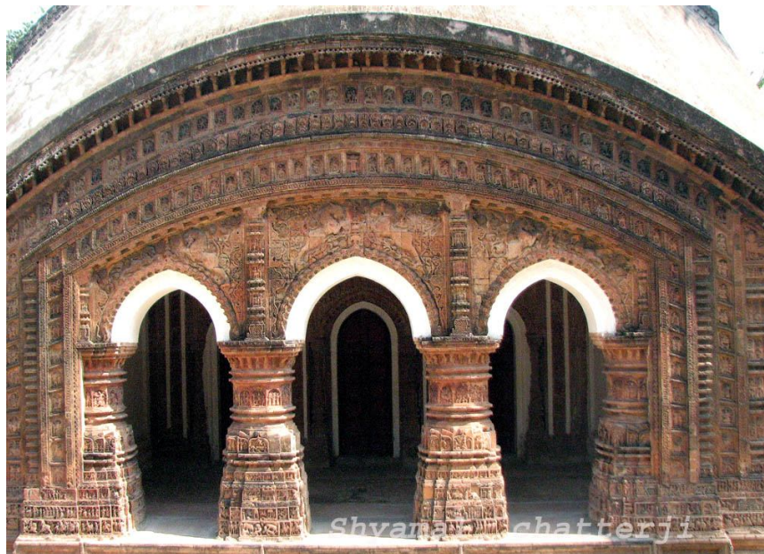
Gangeswar temple, built in 1753 AD, is of Jor-Bangla construction. Major terracotta works have been crafted artistically on the pillars at the entrance and lower panels.
