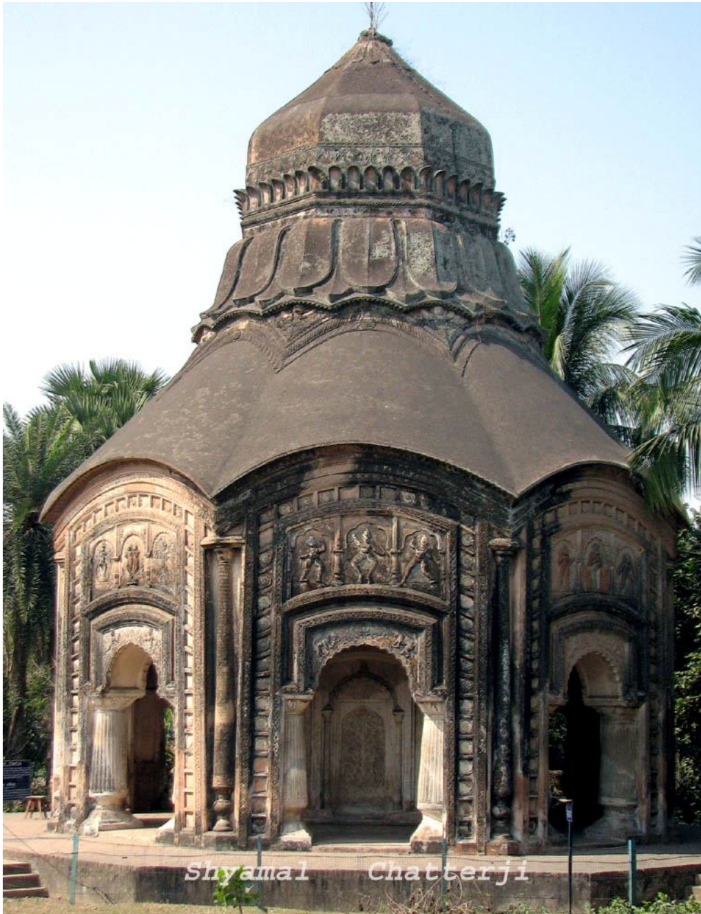
Tallest lime and mortar temple at Baronagar, Built in 1755 AD by Rani Bhavani's daughter Tarasundari. Inverted lotus-like dome of this 18 M tall temple and a circular corridor around the inner sanctum are note-worthy features. Human figures on the outer facade are average. The floral motifs on the outer wall of inner sanctum are excellent.
