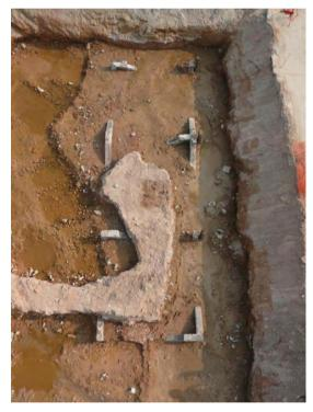
Figure C24 Top View of Landing Steps (wide portion) and Supporting Pillars (narrow portion) of Former Kowloon City Pier
