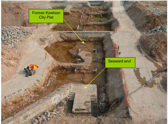
Figure 23 Seaward End of Longjin Bridge and Supporting Pillars of Former Kowloon City Pier
