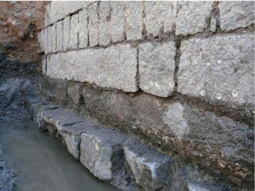
Figure 75 Eastern Side Wall and Footing Stones of Longjin Bridge in T3b
