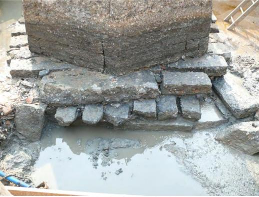
Figure C12 Three Layers of Footing Stones of SP6 (View From East)
