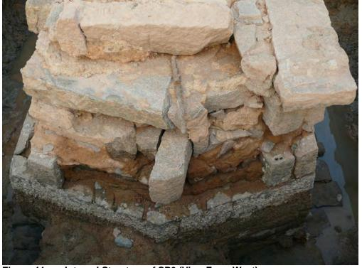
Figure 44 Internal Structure of SP6 (View From West)
