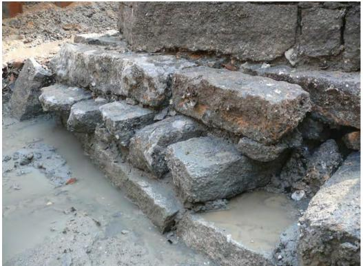
Figure C13 Close-up of Footing Stones of SP6
