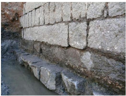
Figure C18 Eastern Side Wall and Footing Stones of Longjin Bridge in T3b
