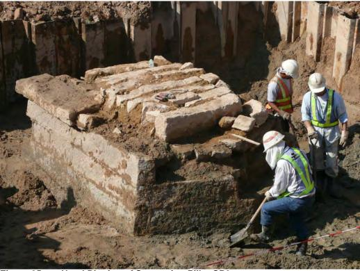
Figure 35 Hand Digging of Supporting Pillar SP6
