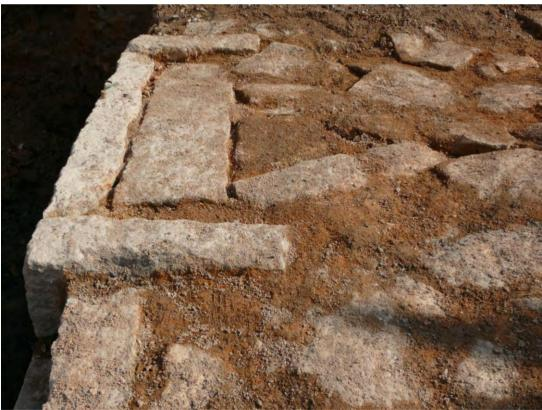
Figure C16 Close-up of Granite Blocks Bonded Together by Sandy Mortar
