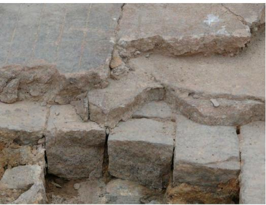
Figure 30 Three Layers of Seaward End of Longjin Bridge
