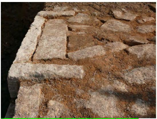
Figure 73 Close-up of Granite Blocks Bonded Together by Sandy Mortar
