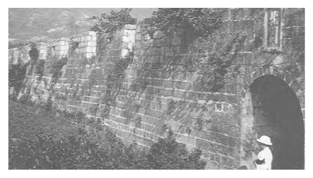
Figure 108 Stone Block Arrangement of Northern Wall of Kowloon Walled City
