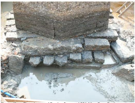
Figure 47 Three Layers of Footing Stones of SP6 (View From East)
