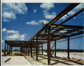
Key factor in concourse design was use of J&L 14-inch Light Beams as purlins. Span between rigid bents varies from 19' 7" to 24' 0". Formed metal decking, which supports insulation and built-up roofing material, is welded to the purlins. Purlins and girders also support a maze of concealed piping.
