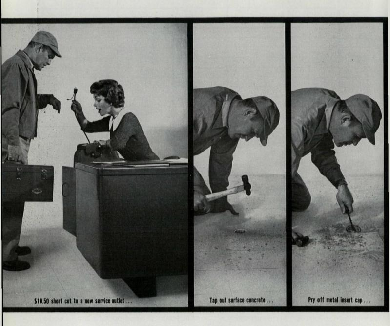
\$10.50 worth of tangible savings every time a new service outlet is installed—complete wiring flexibility for the life of the building... that's where the benefits of an E/R (Electrically Ready) Cofar floor system pay off. Optional factory-installed pre-set inserts on the E/R Cofar cells are an exclusive Granco feature. Eliminate concrete drilling. No noise. No dust. Speed installation of service outlets even during office hours. Fast! Clean! Economical!
