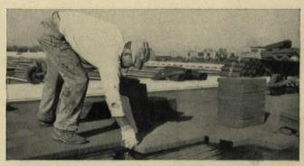
FOAMGLAS Insulation clears the air beneath this roof. Cold outside temperatures contrasting with a hot, humid interior atmosphere, had caused a fog-like condensation. FOAMGLAS roof insulation eliminated the problem. And the incombustibility of FOAMGLAS was an important extra-benefit here.
