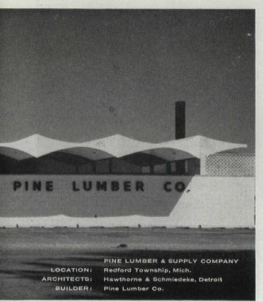
THE AWARD-WINNING DESIGN of this retail lumber showroom is another example of the striking new architectural forms possible with fir plywood, at no sacrifice—in fact, with a gain —in structural strength and integrity.
