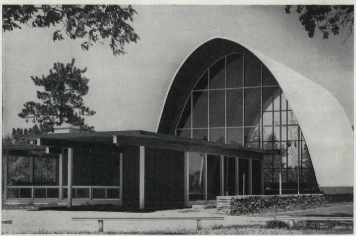
Gracefully bowed laminated beams supporting a parabolic arch, spacious wood-framed glass areas at either end—all combine to create a wide-open setting for a unique treatment of the crucifix. Note how simplicity of design dramatically demonstrates wood's quality throughout this unusual house of worship. Architect: Orus O. Eash.
