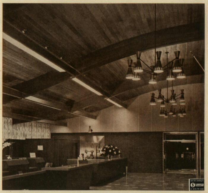
The ability of glued laminated timbers to be formed in almost any desired shape provides an ideal combination
