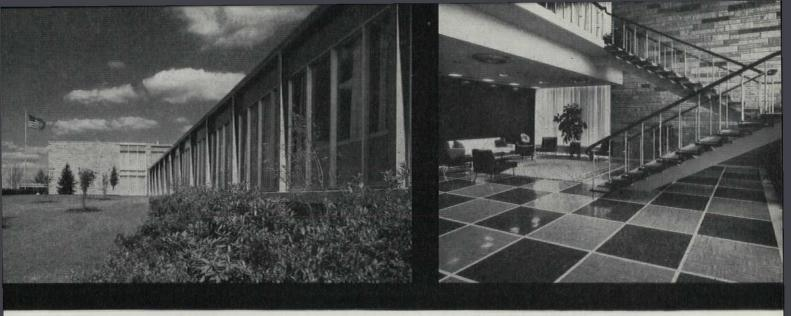
Colorful curtain walls make an eye-appealing exterior. Porcelain-enameled steel panels are blue, steel columns and beams are red.
