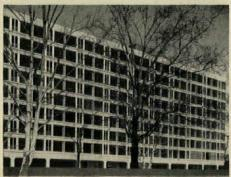
Plaza" ultimately will include four such apartment structures for a total of 512 units, a 17-store shopping center, and a community plaza. The buildings, designed by I. M. Pei & Associates, are of reinforced-concrete construction with windows almost floor to ceiling. An in-swinging, railed window in each room gives the feel of a balcony. At the ground level, each building has a glass-enclosed lobby surrounded by a colonnade. Apart-Continued on page 70
