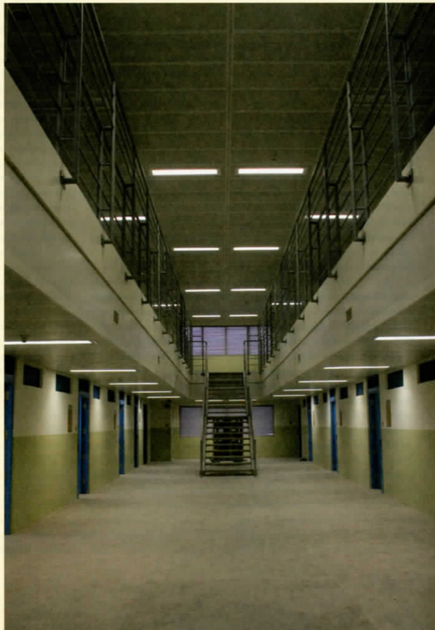
RIGHT The staircase with its open risers is designed to minimise view obstruction.
