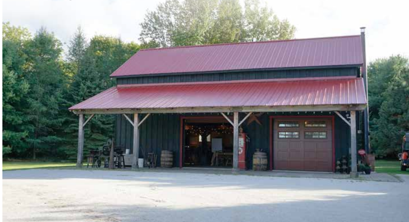
Terry Sheridan rescued the 1860s barn, formerly at the Craigleith Ski Club, from demolition. He tore it down, hauled it to Collingwood, rebuilt and re-purposed it as a studio.
